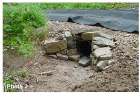
Endwall at pipe outlet.
