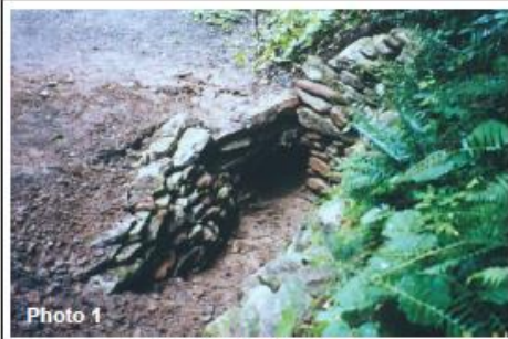
Headwall at pipe inlet.
